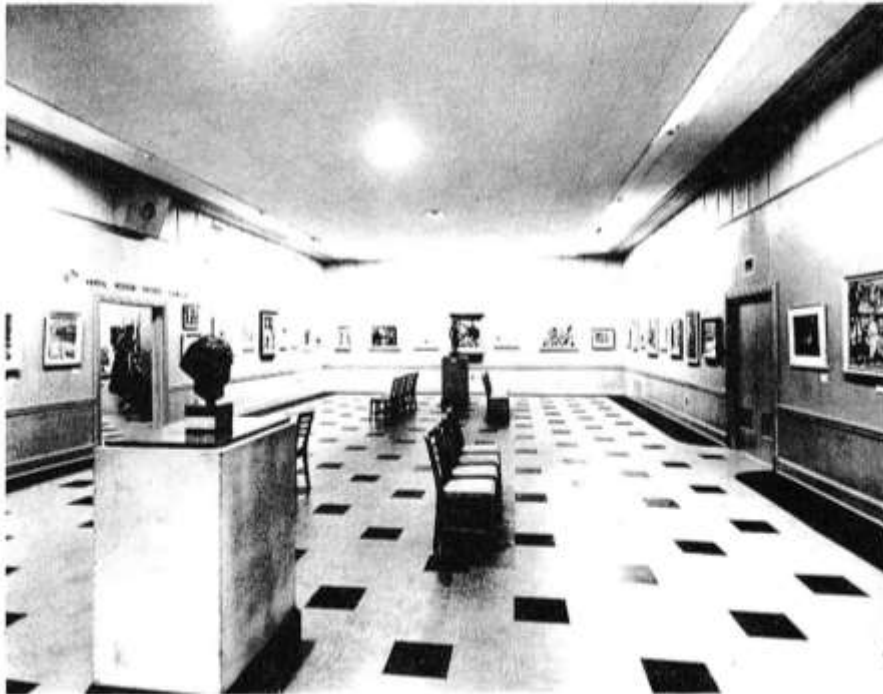
The new central gallery, completed in 1952.
