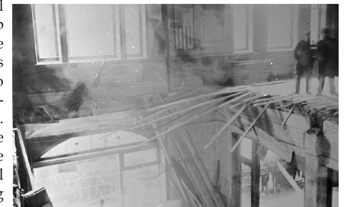
Widely publicized in London, the City Hall collapse shocked the city. However, building regulations did not change until the 20th century with the collapse of the Crystal Hall.
