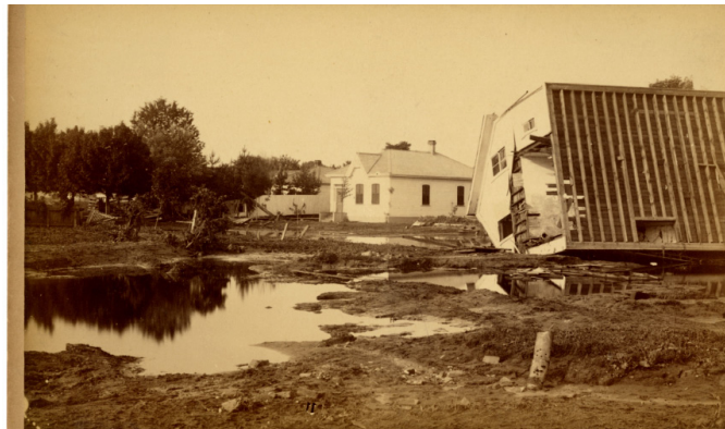
The damage caused by the flood to the city was extreme. As can be seen in this photo, houses completely came off their foundations.
